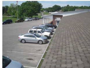
New Gutters & Downspouts
