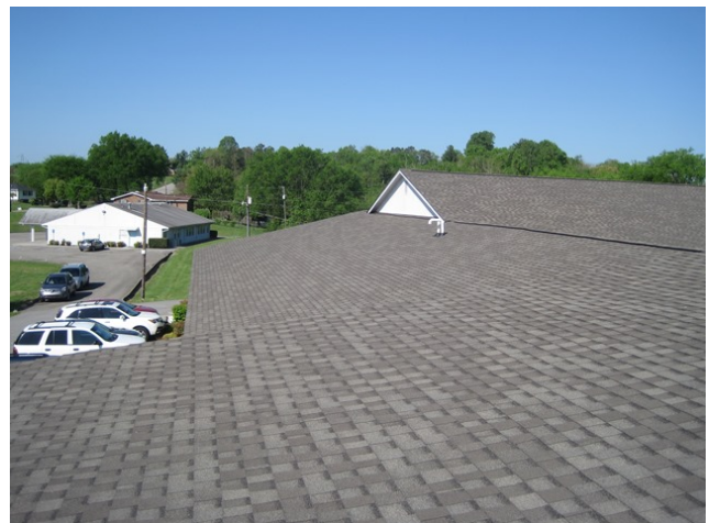
Overall View of the New Shingle Roof
