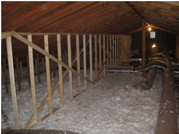
Additional Wood Bracing Added per Code
