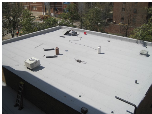
Work in Progress over the Theatre Laboratory
