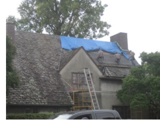
Existing Slate Removal
