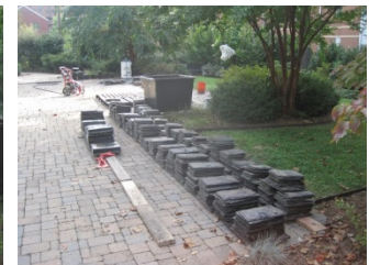
Salvaged Slate to be Reused
