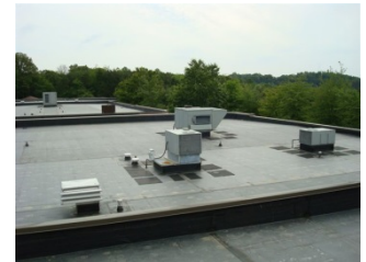
New Adhered EPDM Roof
