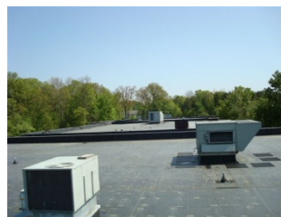
New Adhered EPDM Roof
