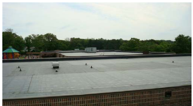
New Fully Adhered 60 Mil Thick EPDM Roof
