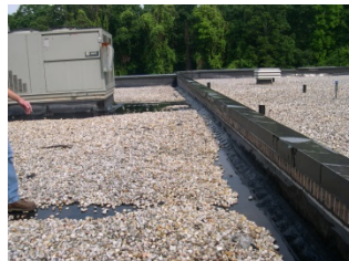
Existing Ballasted EPDM
