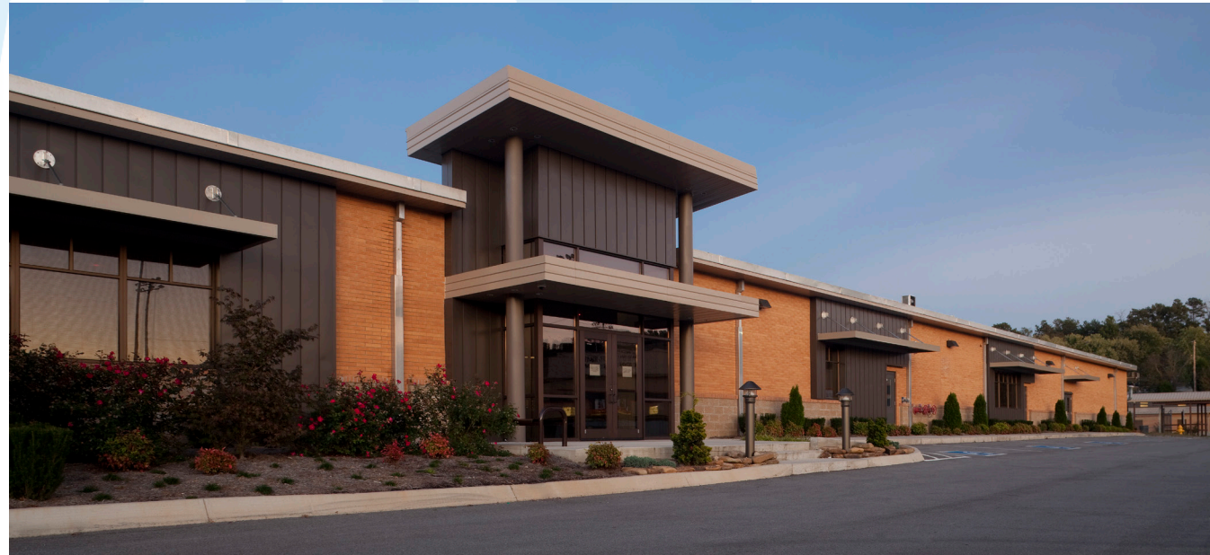
Renovated Vocational Wing of High School
