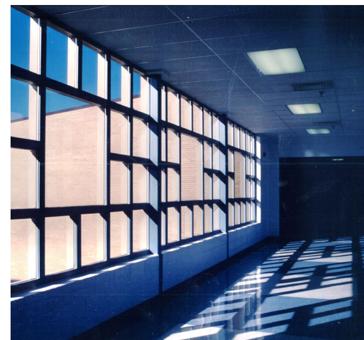
Interior of Pedestrian Bridge
