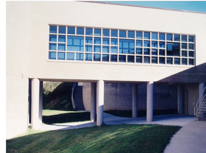
Exterior of Pedestrian Bridge
