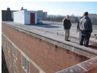
Existing Parapet Wall
