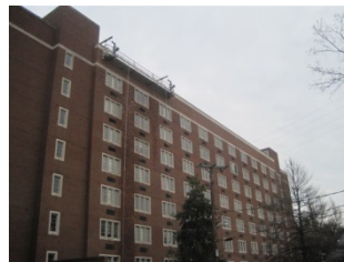
Parapet (Work in Progress)
