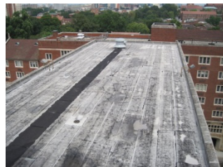
Existing Roofing System
