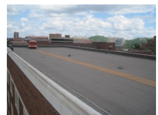
Parapet (New Precast Band)
