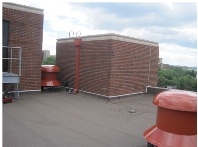
The New 2-Ply Modified Bitumen Roof System (Leak Free)
