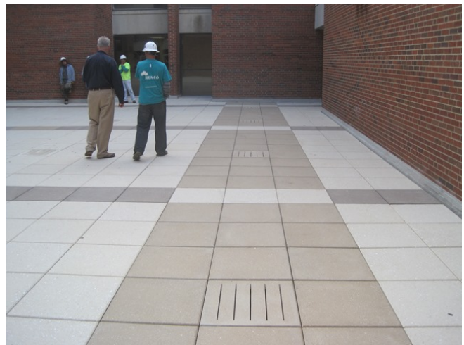
New Courtyard on the North End of Dabney-Buehler Hall
