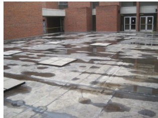
Exist. EPDM Beneath Pavers
