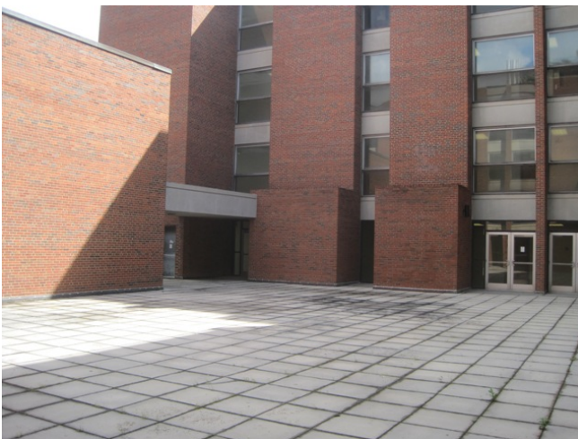
Existing Courtyard on the North End of Dabney-Buehler Hall
