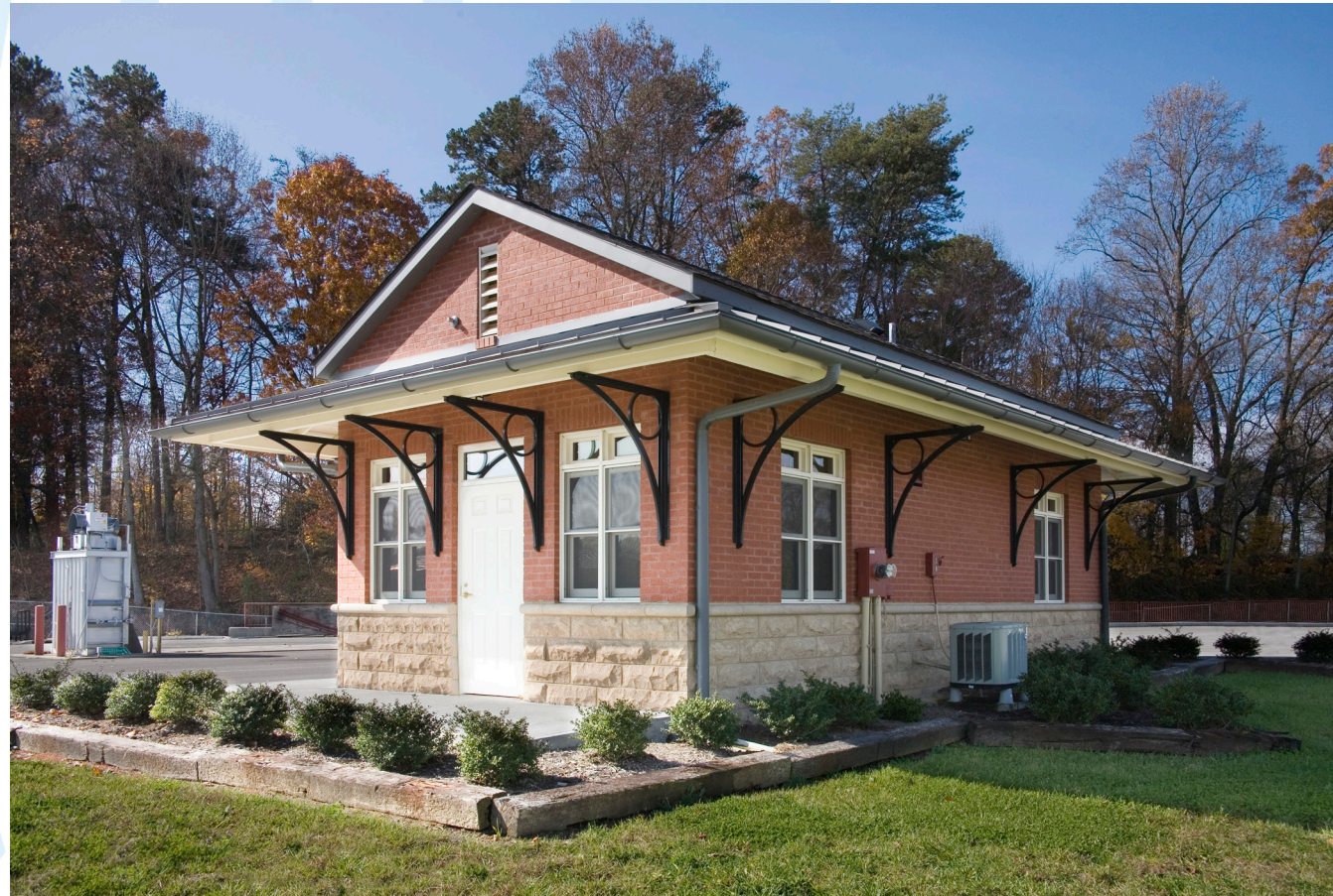
Loudon County Convenience Center
